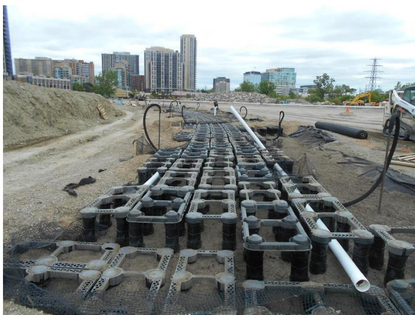
*Figure 13* Installation of DeepRoot Green Infrastructure Silva Cells. Source: DeepRoot.
