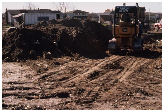
**Figure 5** Construction traffic and soil modification during construction activities can result in soil compaction, which can constrain the growth of newly planted trees. Source: Glen Lumis.
