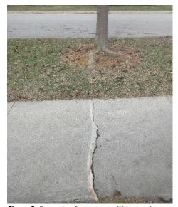
**Figure 2** Example of a tree root lifting and cracking a sidewalk.
