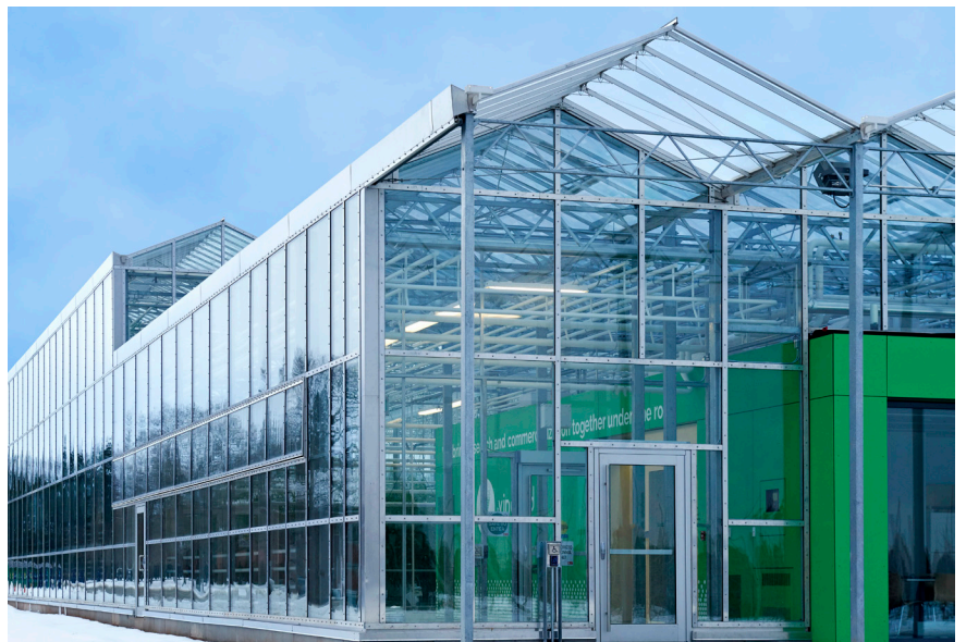
Vineland's new Greenhouse Technology Centre.
