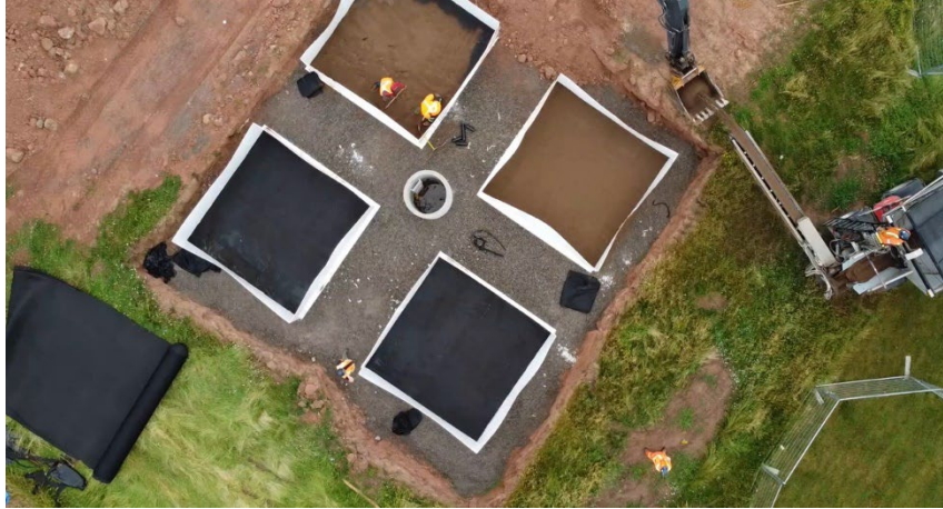
Phase one construction of the new Vineland's TreeCulture Research Park.
